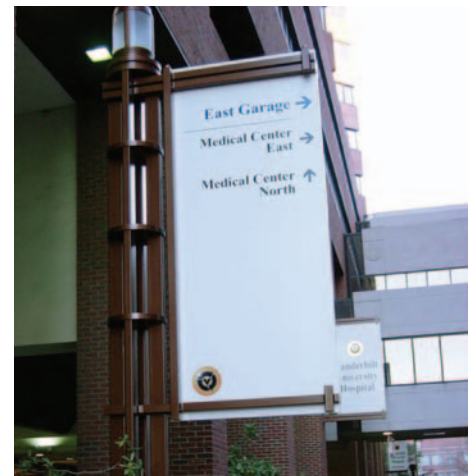
▲ AGI used structural adhesives to construct metal frames and to attach materials to those frames for signage at Vanderbilt University, Nashville.
