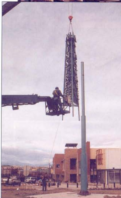
An 80' hydraulic crane lifted the tower sign up and slipped it over a 40' pole, bolted into the concrete base.
