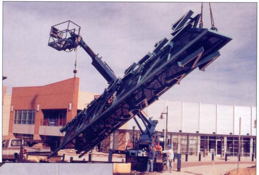
An 80' hydraulic crane lifted the tower sign up and slipped it over a 40' pole, bolted into the concrete base.
